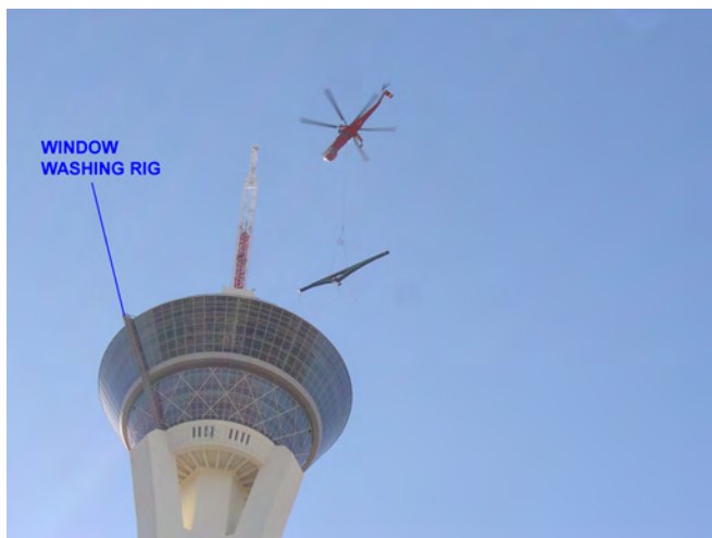
Figure 19. A portion of the X-Scream is lifted into place by helicopter.
