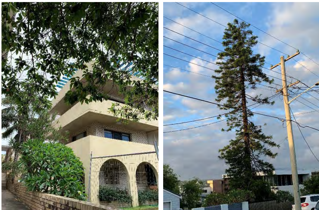
Figure 5: Unit block on Pacific Pde lost its roof yet suffered no damage at ground level (L). Branches snapped from the central 1/3 of a Norfolk Island Pine (R).
